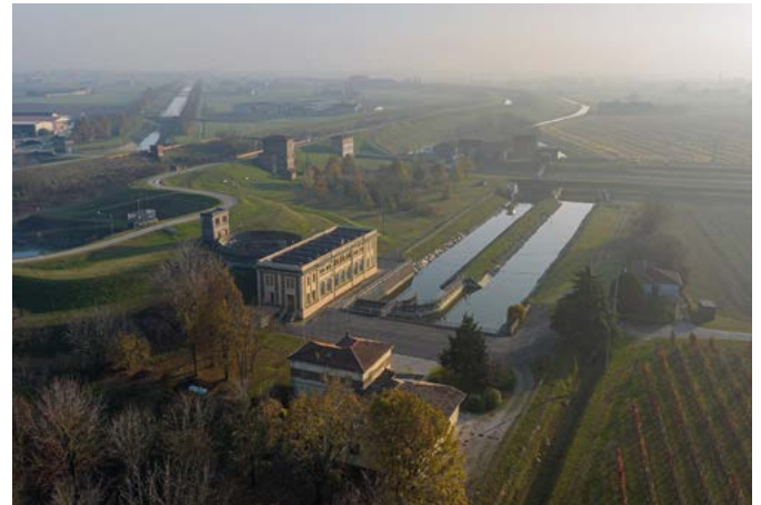
TORRIONE WATER PUMPING PLANT
